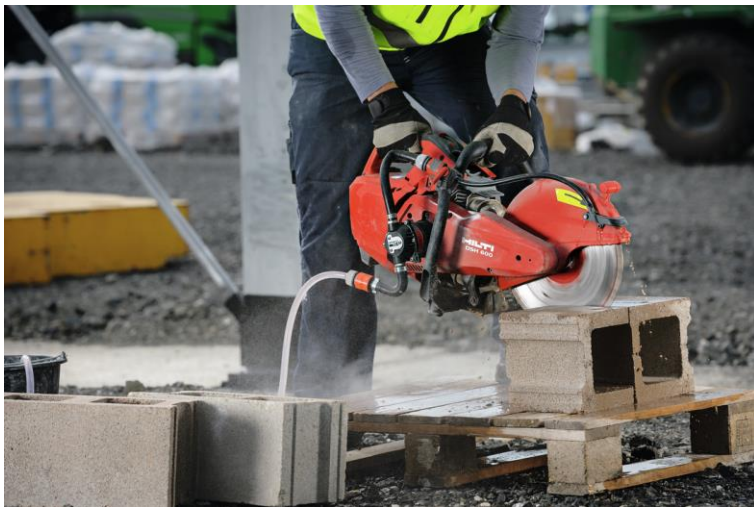
Figure 2: on tool water suppression (source: Hilti Australia)
